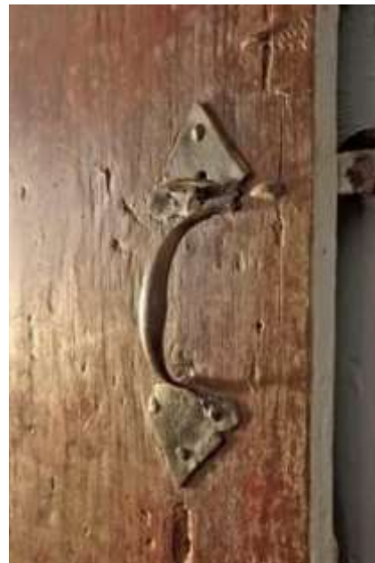
Figure 43: Wrought-iron hardware and hand-forged nails on this distressed wooden door show the soft patina of time???more than 280 years o
